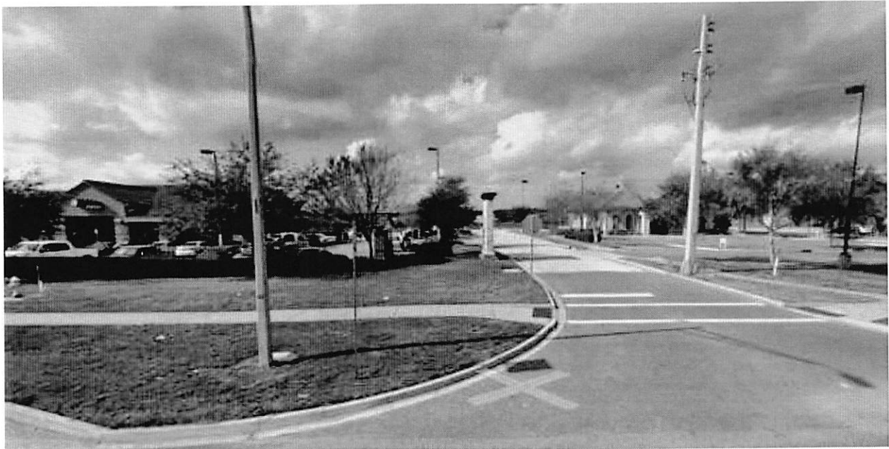
Adjoining commercial along Kernan Boulevard South (subject property behind) Source: Google StreetView Date: 08.03.2017
